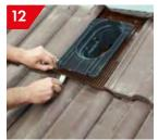
Once Tile Vent is dressed to the tile, clip the cap onto the base securely. Carry on tiling as normal
