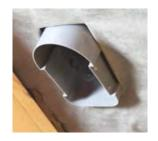
If the vent tile is being used for roofspace ventilation only, the spigot on the back of the vent tile should be left open as shown'
